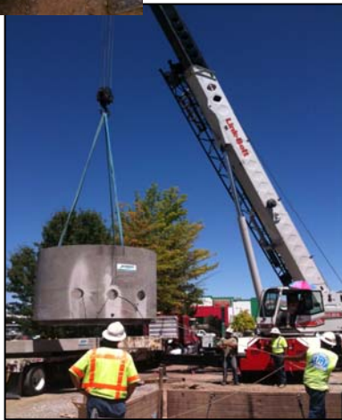
Installation of pump station component, Snider Way
